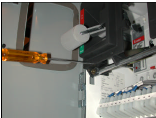
Fig. 25 HMCP Magnetic Adjustment
