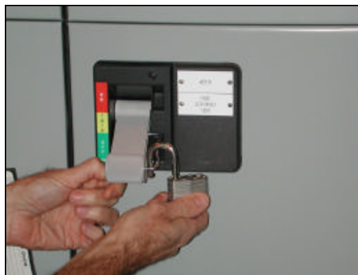
Fig. 34 Locking Out a Disconnect
