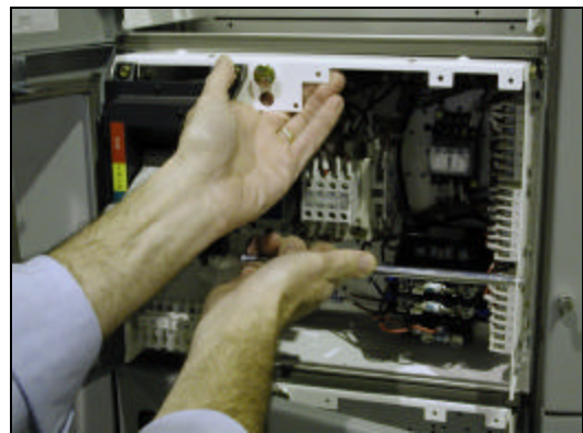
Fig. 28 Withdrawing a Unit
