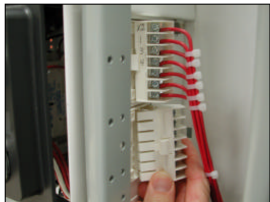
Fig. 27 Disengaging Pull-Apart Terminal Blocks
