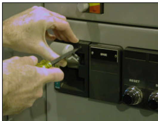
Fig. 33 Defeater Mechanism
