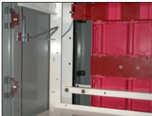
Fig. 31 Shutter Arm Linkage
